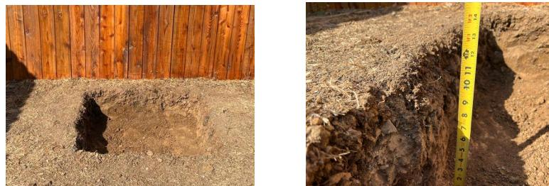
3. Place a thin layer of sand in the bottom of the hole to help level the reservoir and bring the final depth of the hole to 10 inches. This will place the top lip of the reservoir just above the level of the ground (this will ensure no dirt gets into the reservoir during regular use).
